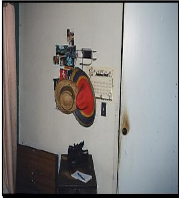
Figure 7 - Interior of patient room, where the door was closed during the fire (NFPA)
